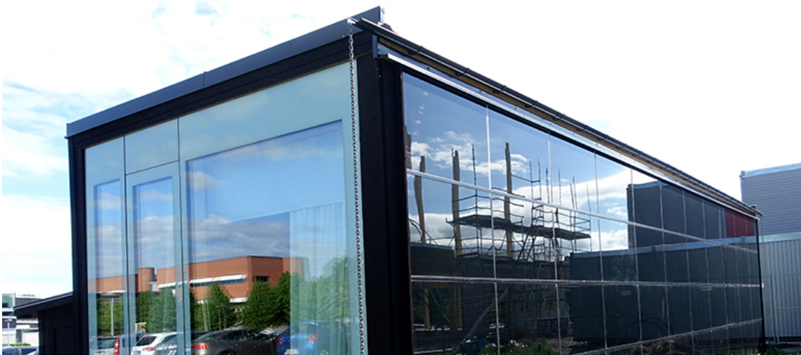
Figure 19: Example of a façade of CIGS PV modules from Solibro, located at the full-scale building prototype of the Innovation Environment Smart Housing Småland www.smarthousing.nu in Växjö.
