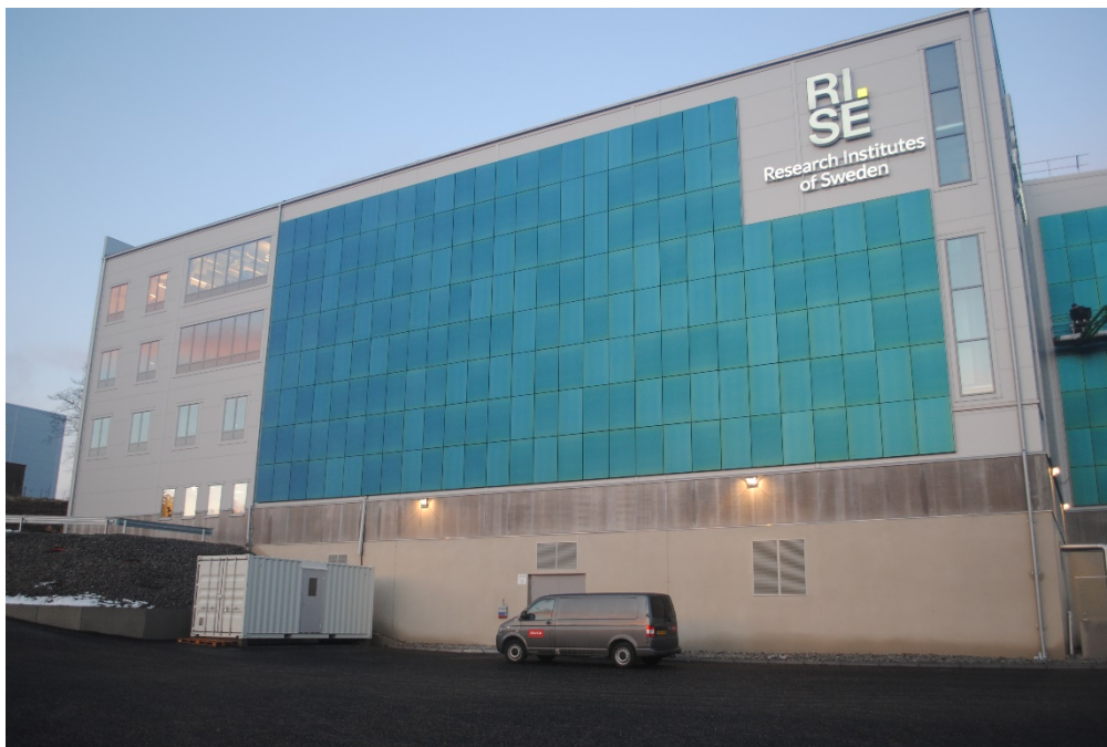
Figure 15: BIPV façade on RISE Awitar Building in Borås. Photo and installation provided by www.SolarLab.dk .
