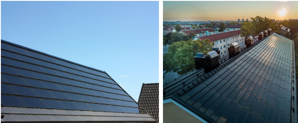
Figure 12: Installations of Left: SolTech RooF and Right: SolTech ShingEl.
