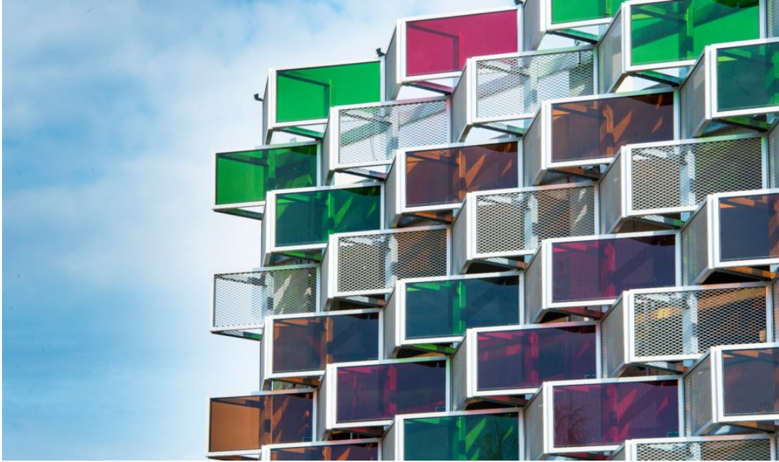
Figure 13: SolTech ST installation at Flustret, Linköping in Sweden. http://www.soltechenergy.com/en/products/soltech-supreme-st-en/
