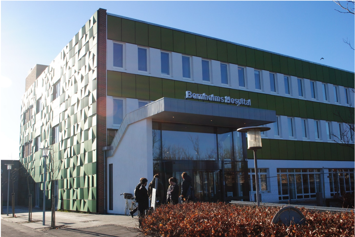
Figure 17: BIPV façade on Bornholms Hospital in Rønne, Bornholm. Photo and installation provided by www.SolarLab.dk .
