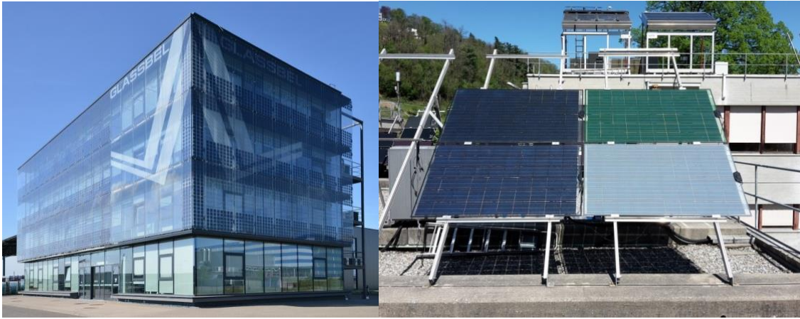
Figure 28: SmartFlex modules, www.smartflex-solarfacades.eu/project , (Source: SUPSI, modules manufactured by Viasolis and Glassbel)
