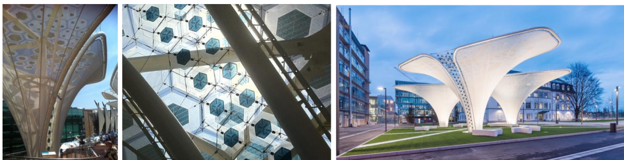
Figure 15: Example of leaf-integrated OPV modules, pioneering organic photovoltaic technology in the German pavilion, Schmidhuber Architects, Expo Milan 2015, Italy (left and centre:© Cristina Polo López). The OPV Solar Trees now stand in the redesigned entrance area of Merck KGaA in Darmstadt (right © Merck KGaA)
