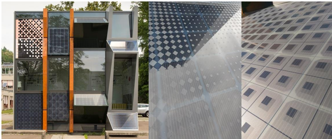
Figure 27: Façade mock-up developed within the EU-funded Construct-PV FP7 project ( http://www.constructpv.eu ). The mock-up demonstrates variants and possibilities in terms of architectural and technological design/manufacturing of BIPV systems for the building envelope (Source: SUPSI)
