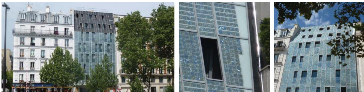
Figure 10: Building with BIPV façade with coloured c-Si cells (LOF), project Fondation Abbé Pierre in Paris ( www.ertex-solar.at/produkte/referenzen );©ertex-solar
