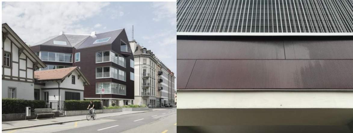
Figure 26: Digital ceramic print on glass/glass BIPV modules with various dimensions developed by ertex solar GmbH. Multi-family building Wohnhaus Solaris, Zürich (CH) (Source: HBF AG)
