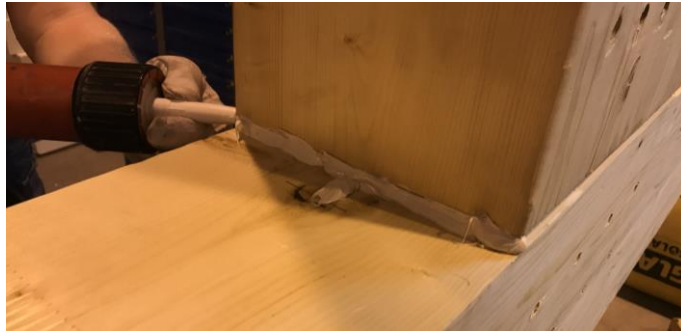
Figure 9: outer 2cm wide fire Sealant in the gap of the connection
